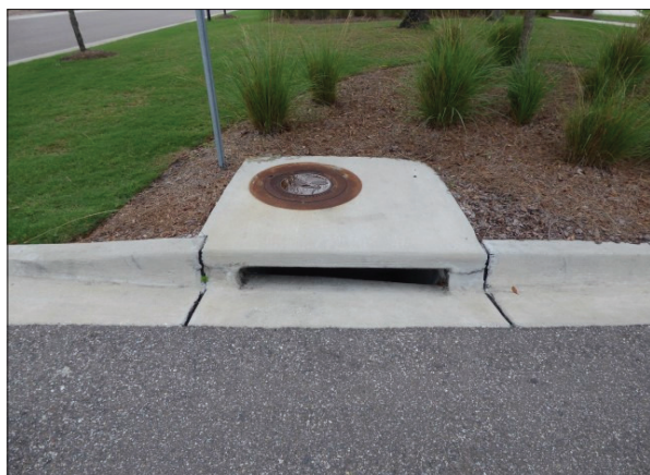
Stormwater Drainage Curb Inlet
