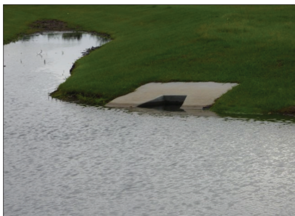
Stormwater Drainage Mitered End Section
