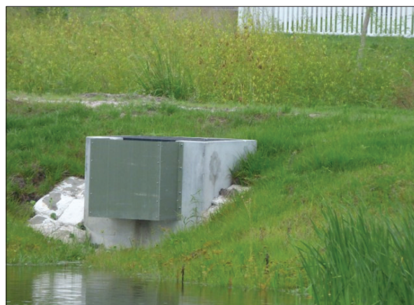
Stormwater Drainage Control Structure
